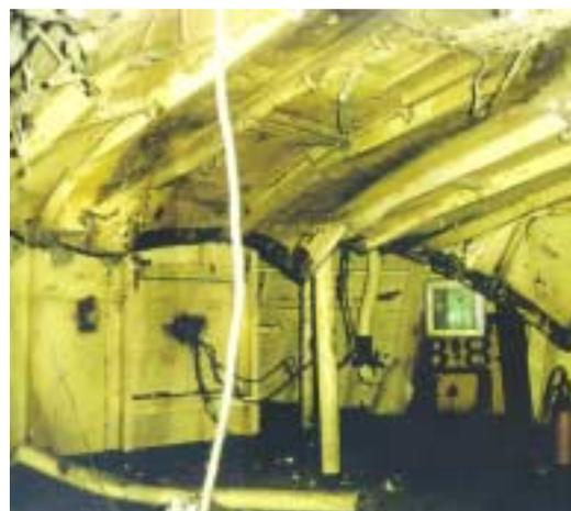
**Figure 14 Failed conventional WT Bulkhead during the Roofdier Trials**
